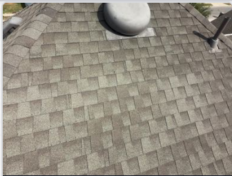
EXHIBIT D FIELD PHOTOGRAPH
